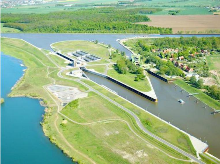
The water-saving lock Rothensee and the longest canal bridge in Europe (918 m) which spans the river Elbe, the double ship lift Hohenwarthe and the connecting canals are all part of a gigantic building project to connect the waterways of Hannover, Magdeburg and Berlin.
